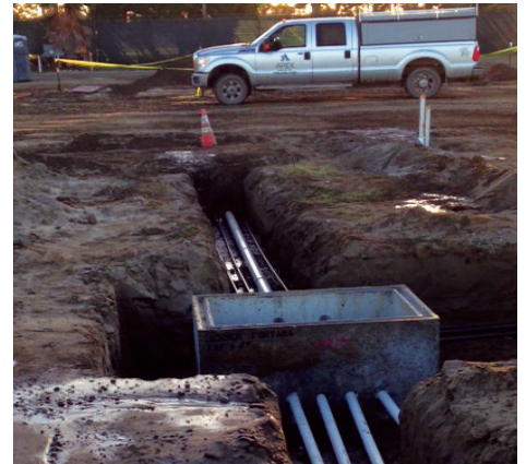
Installation of Remediation Piping
