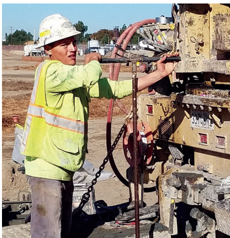
Installation of Remediation Wells
